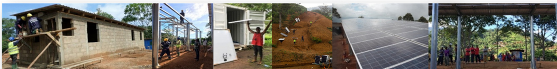
2017: ENSOL & TTA: Design, Construction, and O&M of 1 Solar PV micro-grids (48 kWp) in Mpale, TZ
