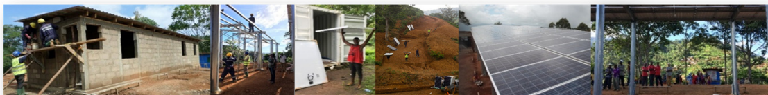
2017: ENSOL & TTA: Design, Construction, and O&M of 1 Solar PV micro-grids (48 kWp) in Mpale, TZ
